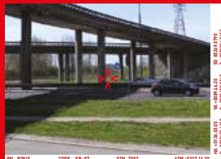
Infrastructure & Road construction
